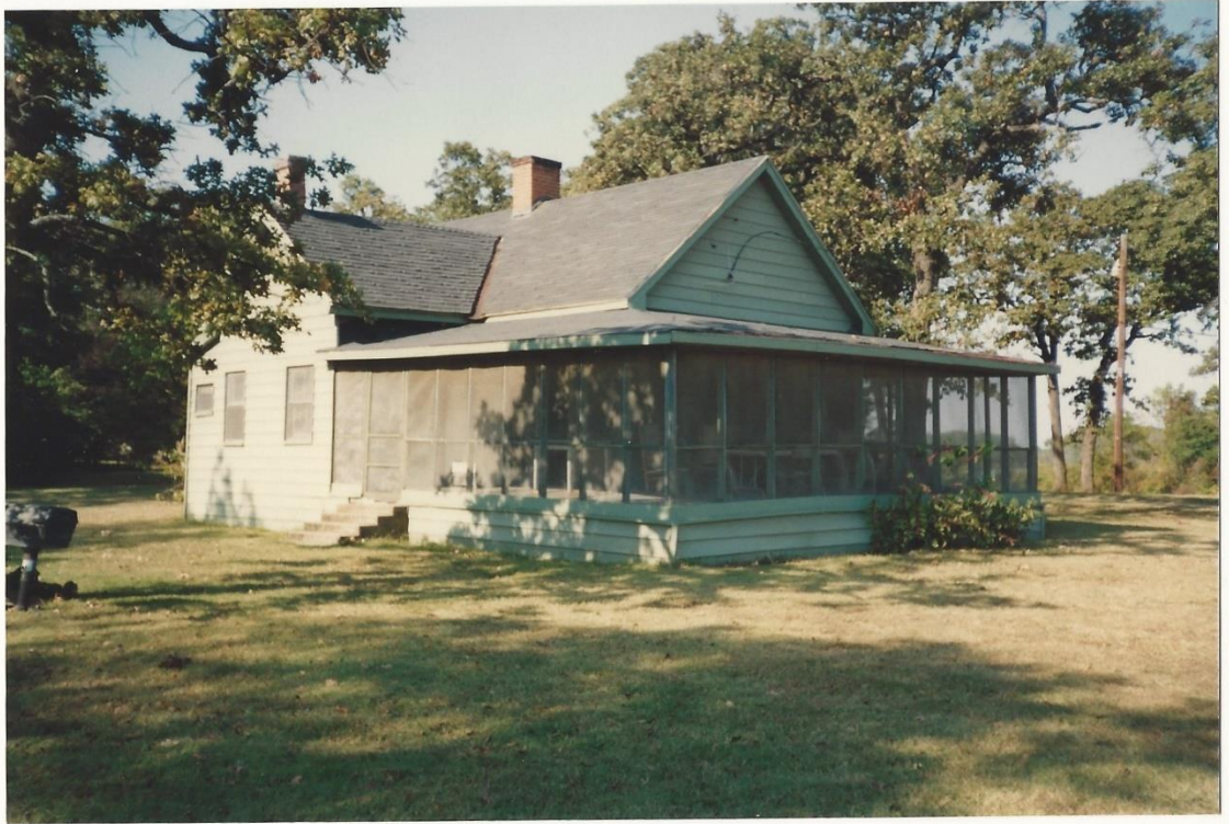
Family cottage (Thomas house) from southwest corner
