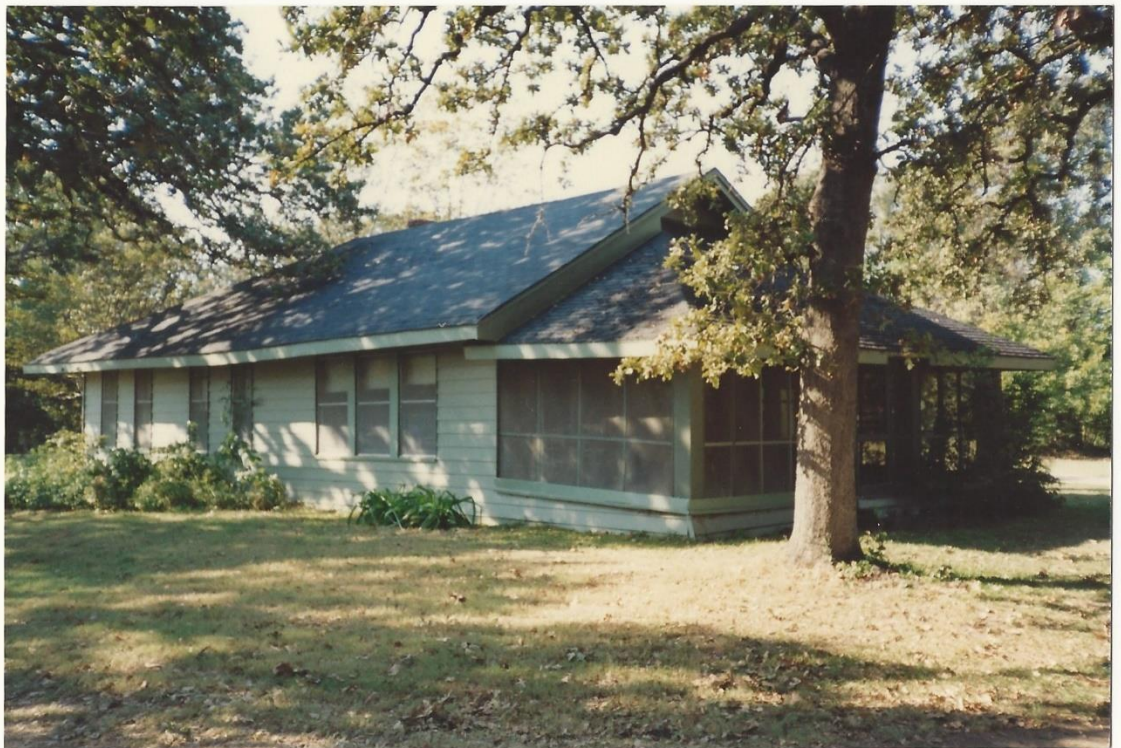
Ladies clubhouse from southeast corner
